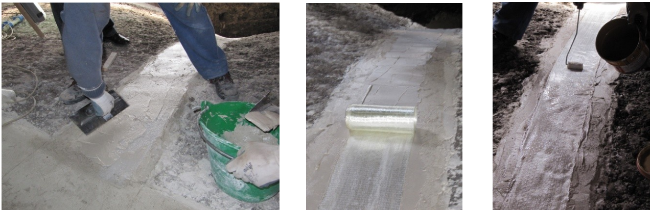
fig. 1.h - Steps of FRP application (strengthening of the vaults of the church “Spirito Santo” in Nicolosi - CT): application on a leveling mortar of a layer of epoxy resin (photo 1), placing of the dry monodirectional glass fabric (photo 2), application by roller brush of a epoxy resin layer (photo 3)
