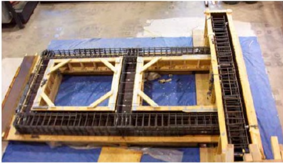
Figure 110 – Full steel and partial formwork assembly [DSV07].
