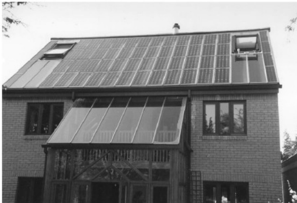
Figure 22 PV roof installation
