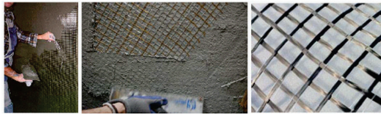
Figure 1.1: FRCM Fibre Reinforced Cementitious Matrix.
